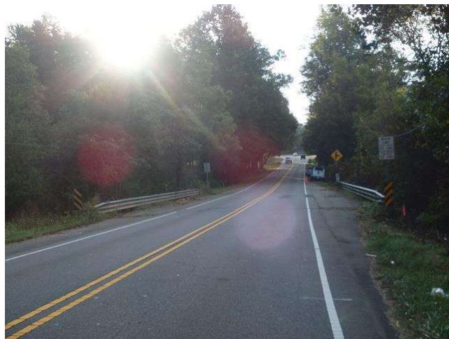
Figure 14 | Robinson Church Road Bridge
