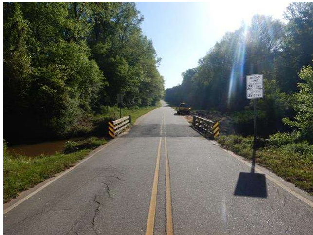
Figure 13 | Lockhart Road Bridge
