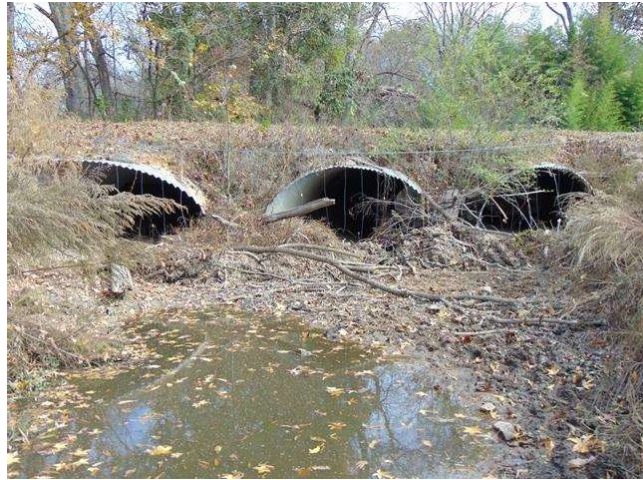
Figure 15 | Austin Grove Road Culvert
