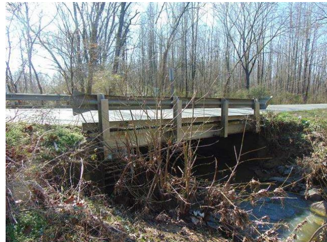
Figure 9 | Monroe-Ansonville Road Bridge
