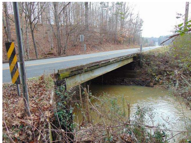
Figure 11 | Shannon Road Bridge
