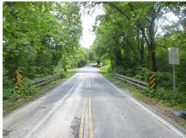
Figure 7 | Peach Orchard Road Bridge
