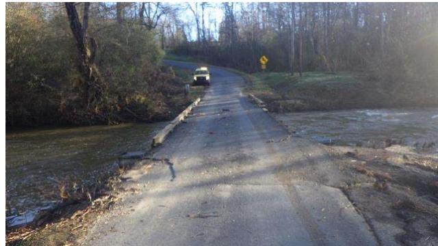
Figure 10 | Bridgeport Road Bridge
