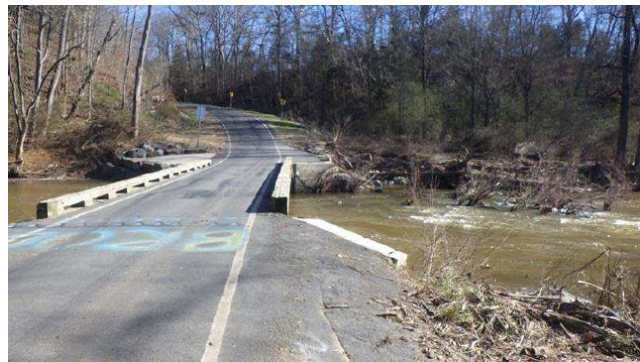
Figure 12 | Booger Hollar Road Bridge
