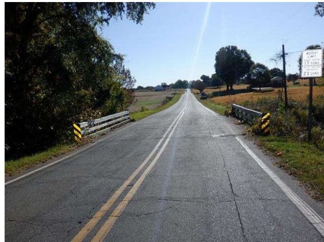
Figure 8 | Stack Road Bridge
